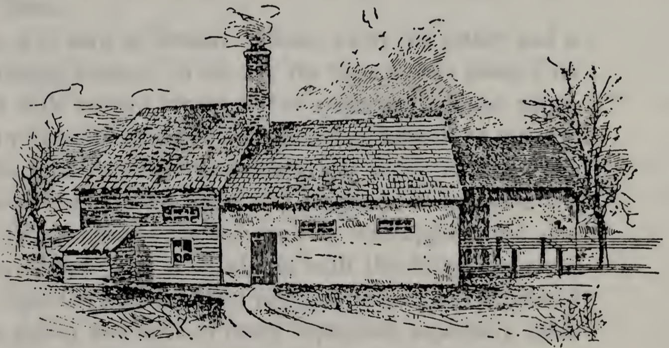
The Original Trenton Plant of the Roebblings in 1849
